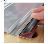
With adhesive side facing main track body, align end of guide strip with end of track and fit into groove. Once positioned correctly, firmly press into set.
